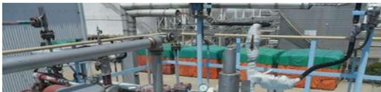
Emergency depressurization (EDP) valve sized to depressurize the system to 50% of the vessel's design pressure in 15 minutes or less (to protect against Bleve)
